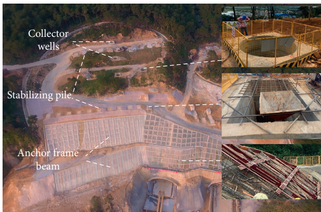
FIGURE 7: Deposit slope after stabilization work completed.
