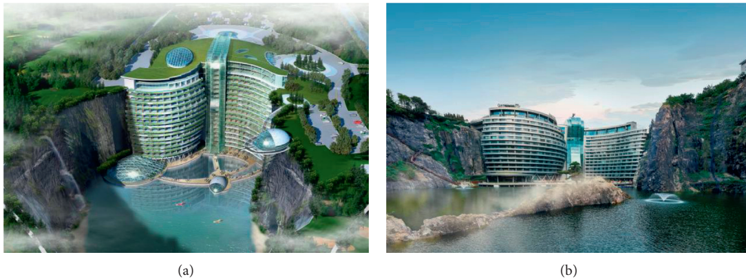
FIGURE 4: 3D rendering and actual photograph of the building. (a) 3D rendering of the building. (b) Actual photograph of the building.
