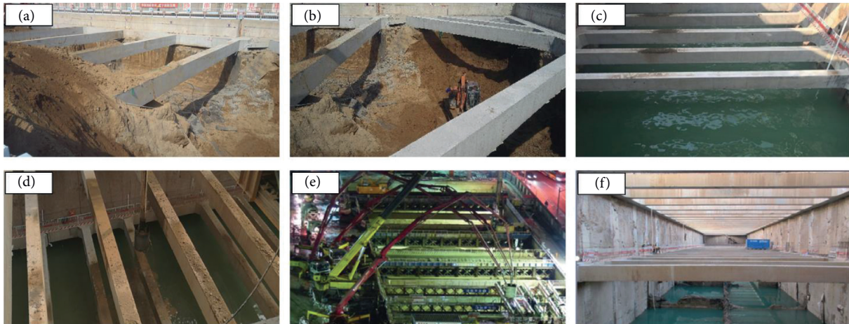
FIGURE 4: Critical steps during excavation for YDM project. (a) Step 1, (b) step 4, (c) step 5, (d) step 6, (e) step 7, and (f) step 8.
