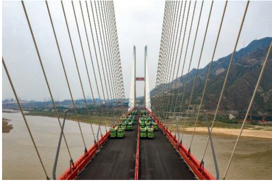
FIGURE 1: Yu Men Kou Huanghe River Bridge.
