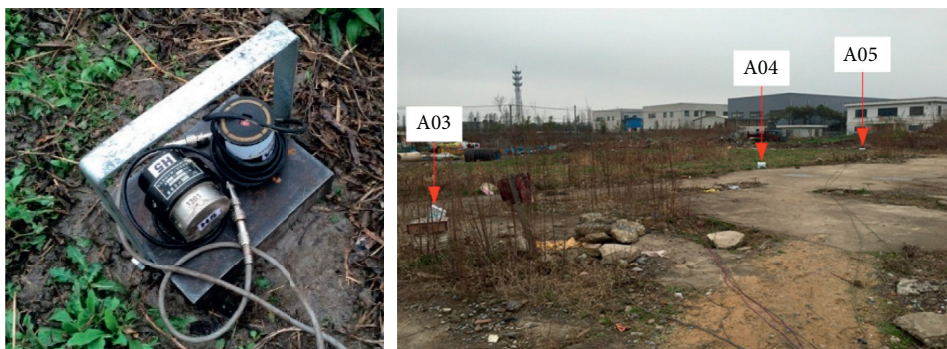
FIGURE 8: Accelerometers installed on the ground surface.
