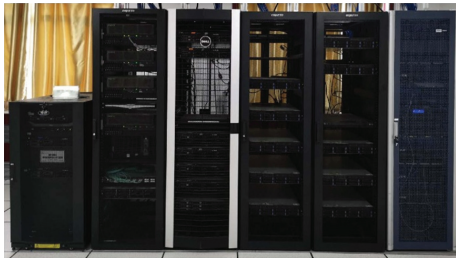
FIGURE 4: Microseismic monitoring center.
