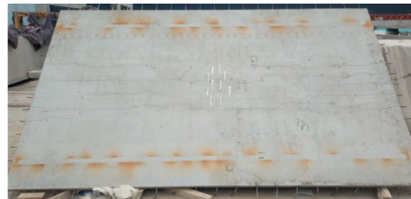
FIGURE 8: The plate cracks of DHB3.
