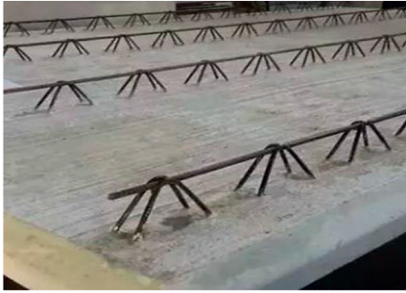
FIGURE 1: The composite slab with steel trusses.
