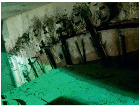
FIGURE 8: Steel sleeve outside the tunnel portal.
