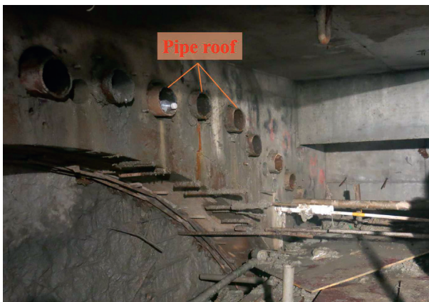
FIGURE 5: Pipe roof installation.
