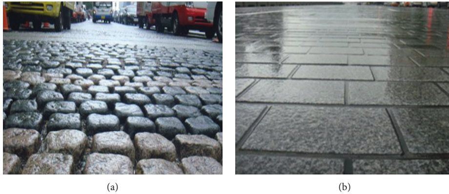
FIGURE 1: Classification of construction methods for stone element pavement. (a) Flexible surface construction (cubes). (b) Rigid surface construction (setts).
