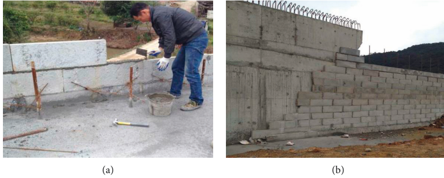
FIGURE 7: (a, b) Cement panel protection.
