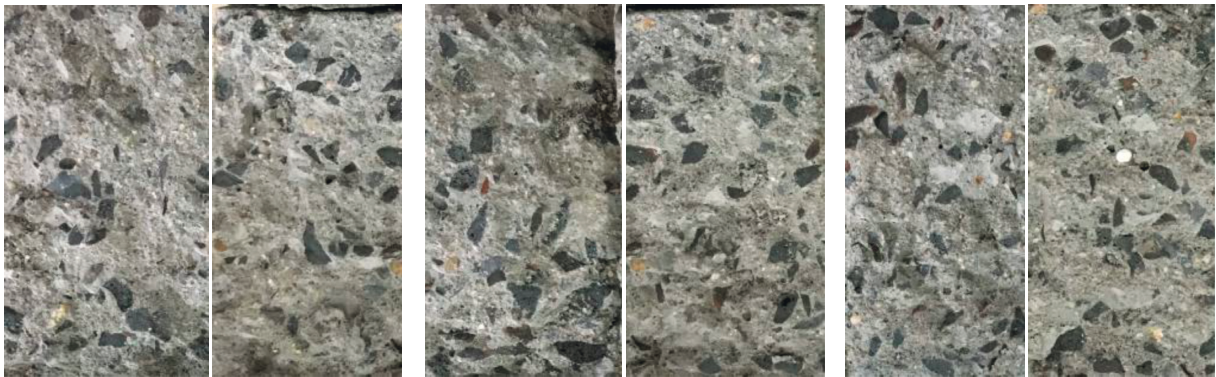
FIGURE 24: Fractured surface in the test.
