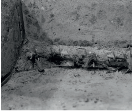
FIGURE 4: Steel-concrete interface for the GPC beam.
