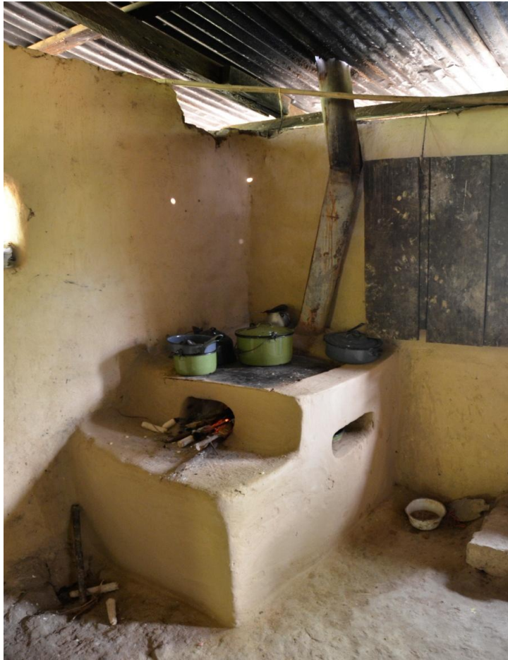
A traditional adobe stove within a home in the village of La Hicaca, Yoro. Of note is the improper installment of the chimney, with a large gap between the chimney and the stove.
