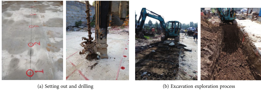
FIGURE 12: Field test of grouting diffusion radius.
