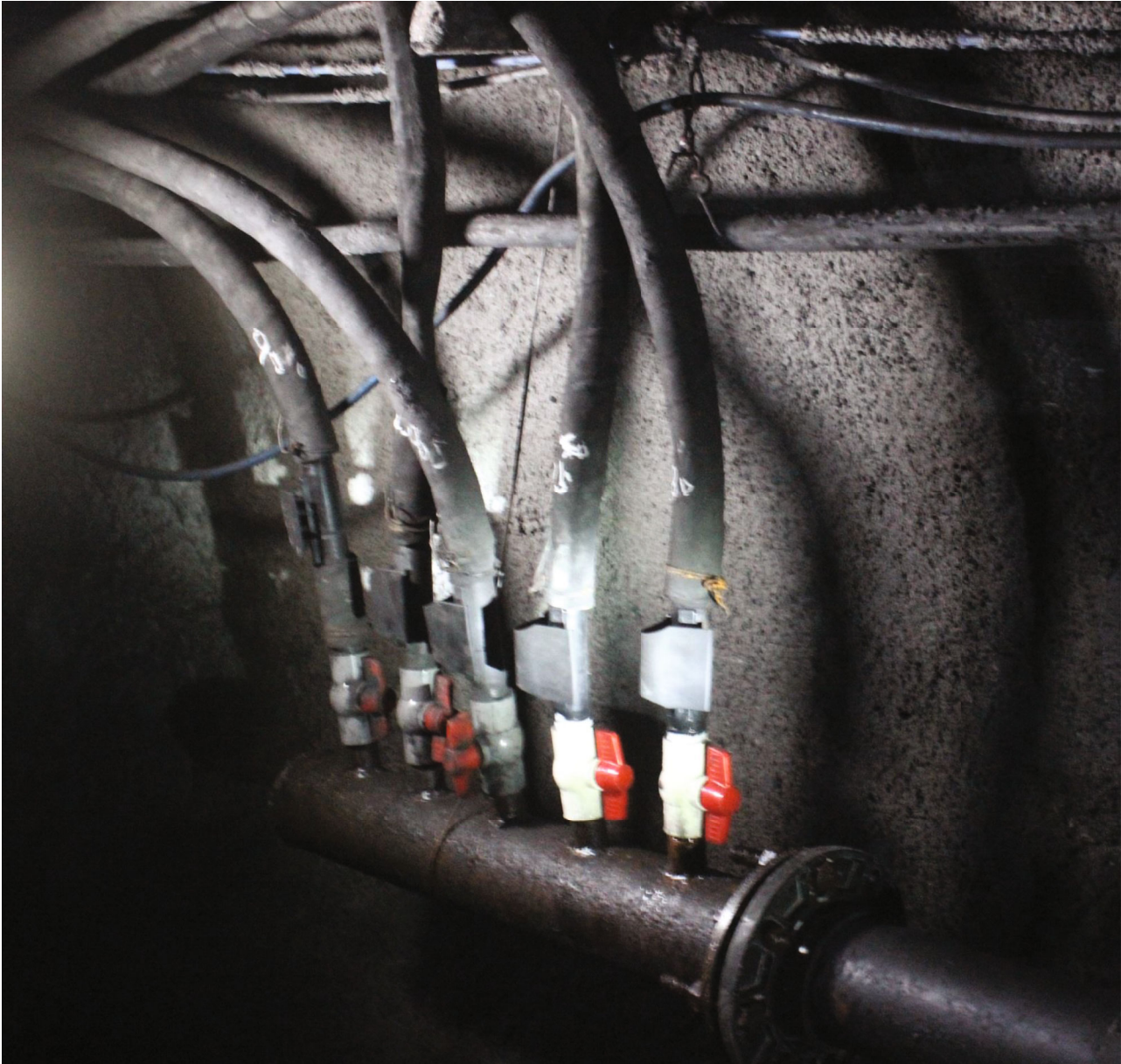
FIGURE 13: Borehole construction and borehole networking.
