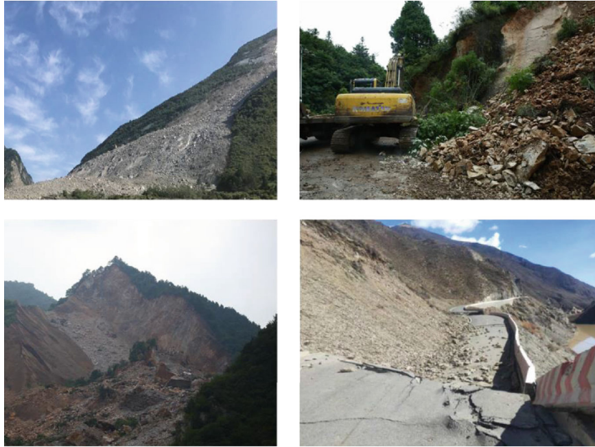
FIGURE 1: Slope instability disaster in China.
