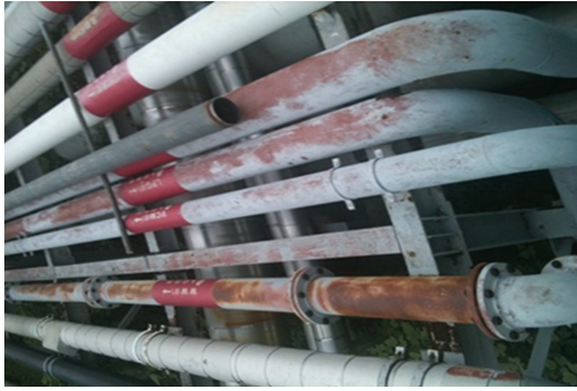
FIGURE 1: A case of the aging and corrosion of pipe racks.
