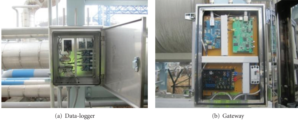
FIGURE 7: Data-logger and gateway of the pipe-rack health monitoring system.
