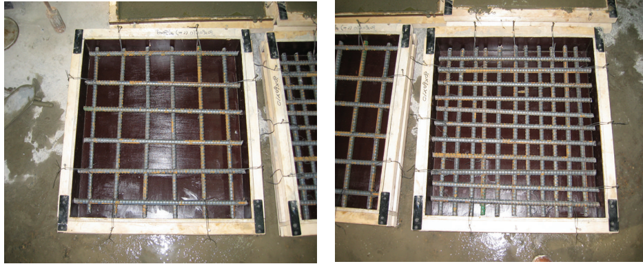
FIGURE 4: Placement of bars (D16@10, D16@5).
