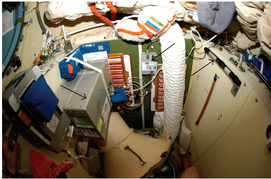
FIGURE 5: EGLE inside the PIRS module of the ISS. Arrows indicate MEB (left), EGLE-MB (front), and EGLE-MH (right).
