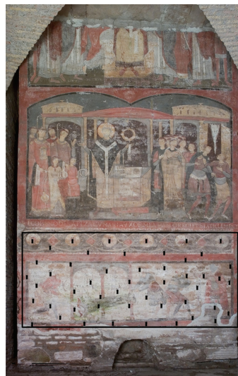
FIGURE 1: St. Clement at mass and the legend of Sisinnius wall painting. The matrix of points where NMR measurements were carried out is also shown. Marked degradation is observed in the framed area whereas the upper part is in a better state of conservation.
