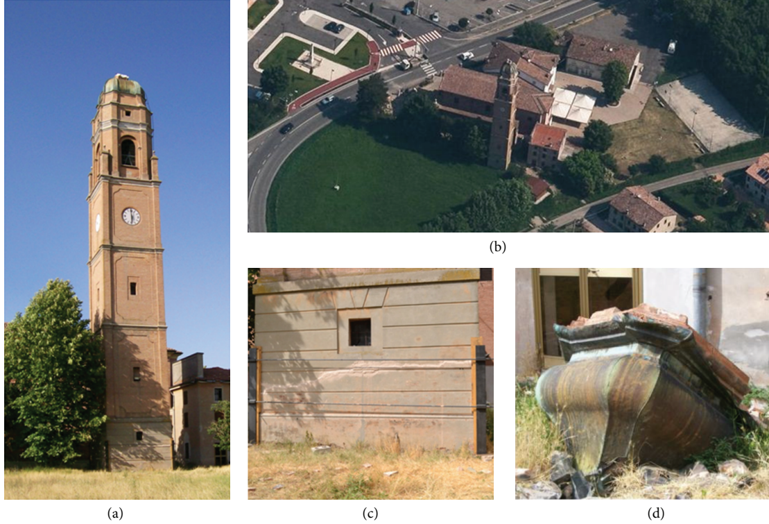
FIGURE 1: Some images of the damaged bell tower. (a) Southwest side of the building. (b) Panoramic view. (c) Cracks at the base of the tower. (d) Collapsed top.
