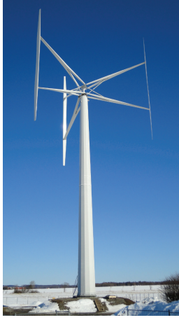
FIGURE 1: A 200 kW prototype H-rotor in Falkenberg, Sweden. The turbine is based on research from Uppsala University [8–10] and is currently one of the largest operating VAWTs in the world.
