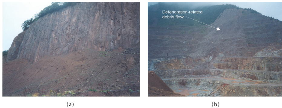
FIGURE 12: Fine debris pile at slope foot (a) and deterioration-related debris flows (b).
