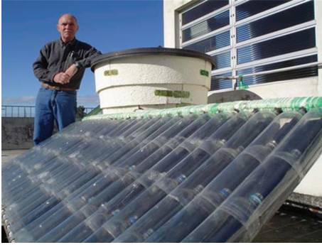
FIGURE 5: View of the tubing collector wrapped with recycled PET bottles.
