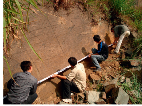
FIGURE 6: The slate rock joint surface.
