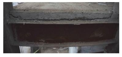
FIGURE 15: Cracks on slab at the second floor.
