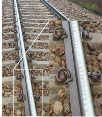
FIGURE 9: Real-life rail corrugation with wavelengths in the interval 4–8 cm occurs due to the accumulation of plastic strains [29].
