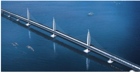
FIGURE 2: Jianghai Shipping Channel Bridge.
