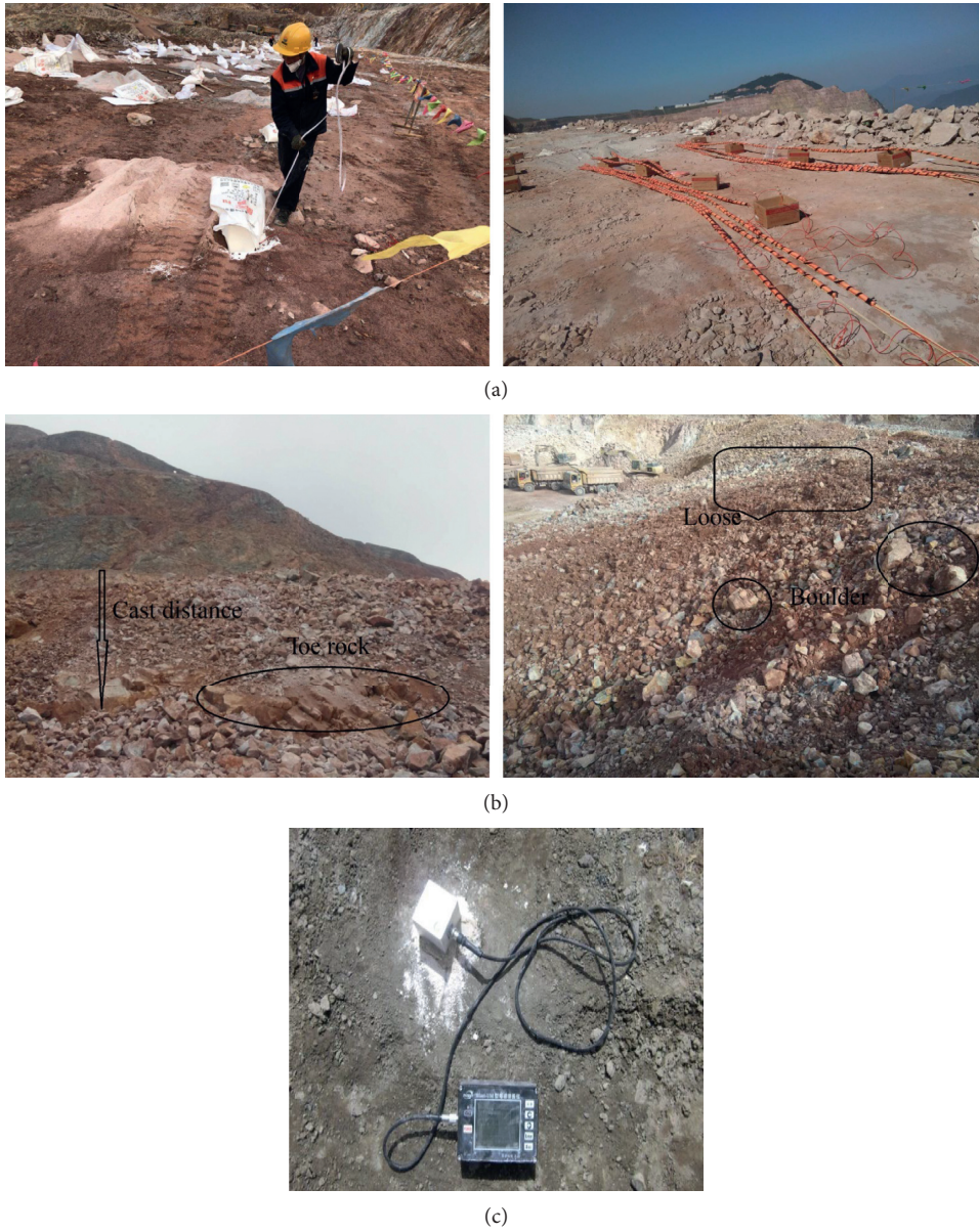
FIGURE 4: Explosion site and the effect after blasting. (a) Before the explosion. (b) After the explosion. (c) Mounting vibrometer.
