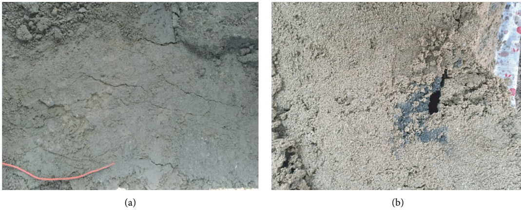
FIGURE 12: Test 3 cracks after blasting. (a) Test 3 cracks formed after blasting. (b) Test 3 cavity zone formed after blasting.
