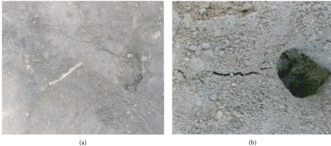
FIGURE 14: Test 4 cracks after blasting. (a) Test 4 cracks formed after blasting. (b) Test 4 cavity zone formed after blasting.
