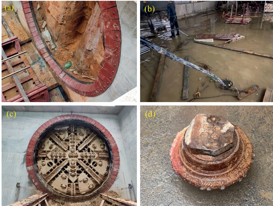
FIGURE 11: Actual excavation situation.
