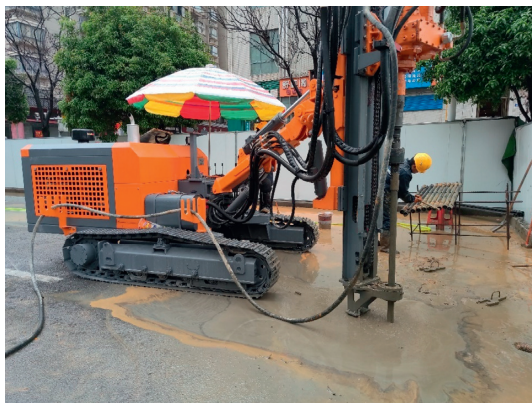
FIGURE 7: Karst cave grouting.
