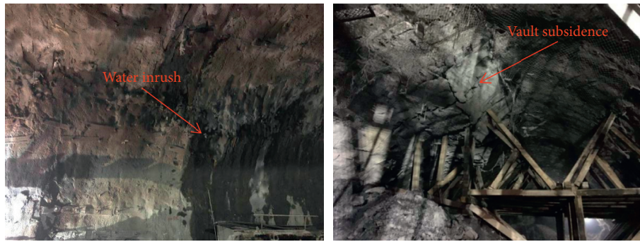
FIGURE 1: Failure characteristics of layered surrounding rocks.
