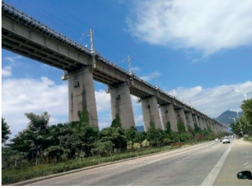
FIGURE 1: HSR bridge (Xiangtang-Putian Railway line).
