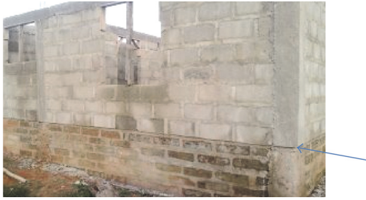
FIGURE 3: Building without floor concrete bed.
