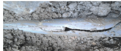
FIGURE 6: A burst PVC pipe beneath paved compound of a house.
