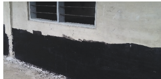
FIGURE 7: Bitumen applied before painting.
