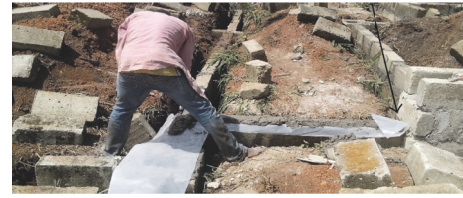
FIGURE 5: Placing of damp-proof material in foundation.
