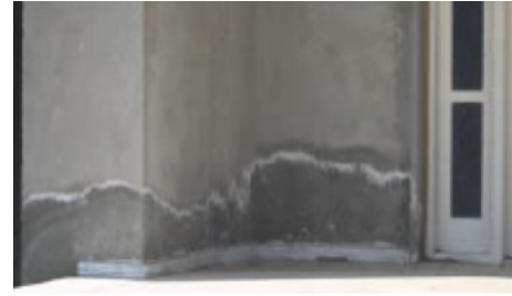
FIGURE 1: Tidal mark on wall in Kumasi.
