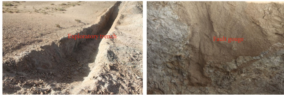
FIGURE 4: Exploratory trench and fault gouge.
