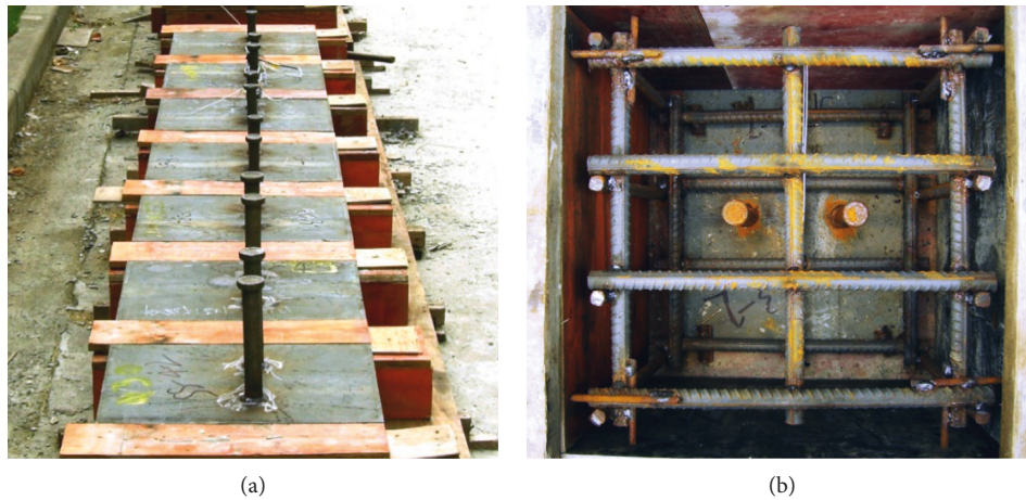
FIGURE 3: Fabrication of push-out specimens.
