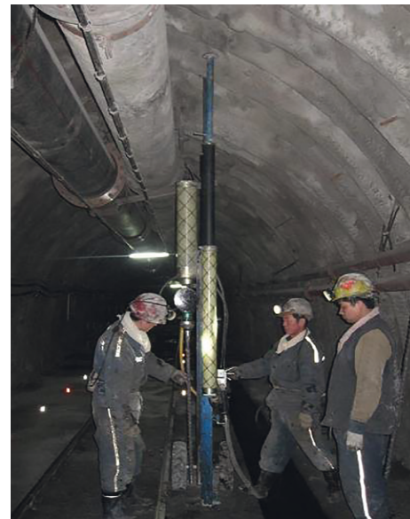
FIGURE 9: Anchor cable rig dedicated by the floor.
