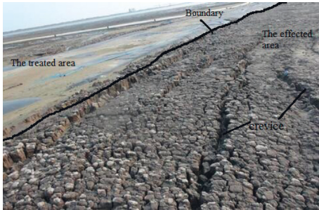
FIGURE 1: Deformation of the soil under vacuum consolidation.
