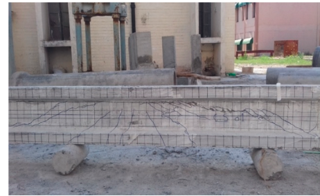
FIGURE 15: Crack patterns of B1-CM.
