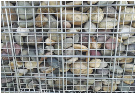
FIGURE 17: Local photos of the pebble iron art fence.
