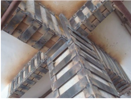
FIGURE 1: Picture of strengthening “angle steel and batten plate.”
