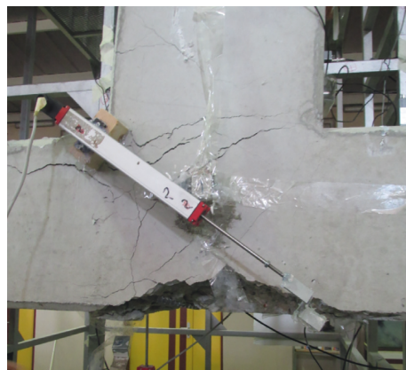
FIGURE 10: Failure of the control sample.
