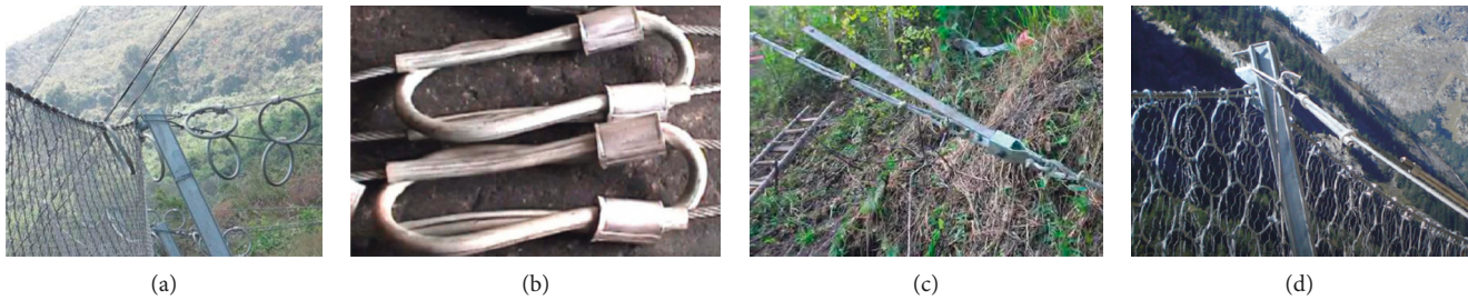
FIGURE 1: The most widely used dissipators in rockfall engineering. (a) Ring brake. (b) Double-U ring brake [6]. (c) U-shape dissipator. (d) Metal-tube-crushing dissipator.
