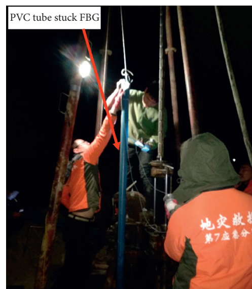
FIGURE 9: Field installation of fiber grating monitoring equipment.
