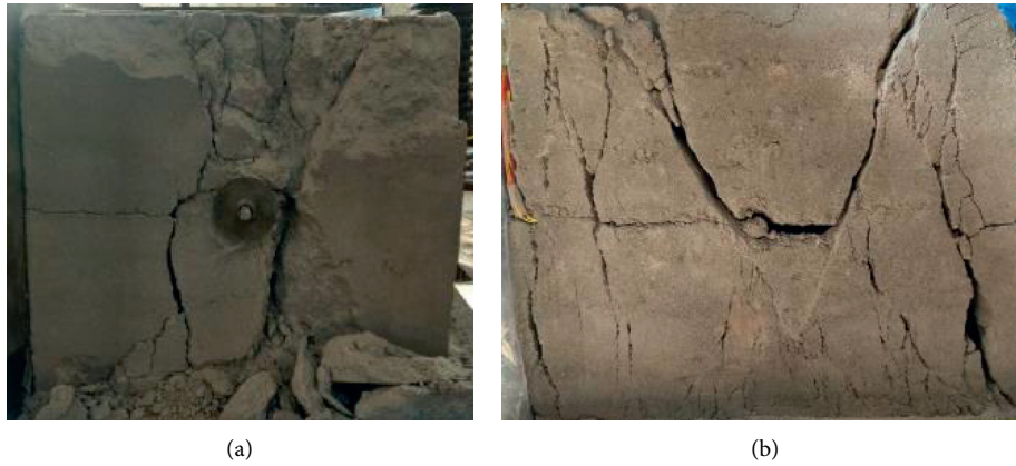
FIGURE 8: Diagram of fragmentation of one rockbolt. (a) Frontal destruction. (b) Side destruction.
