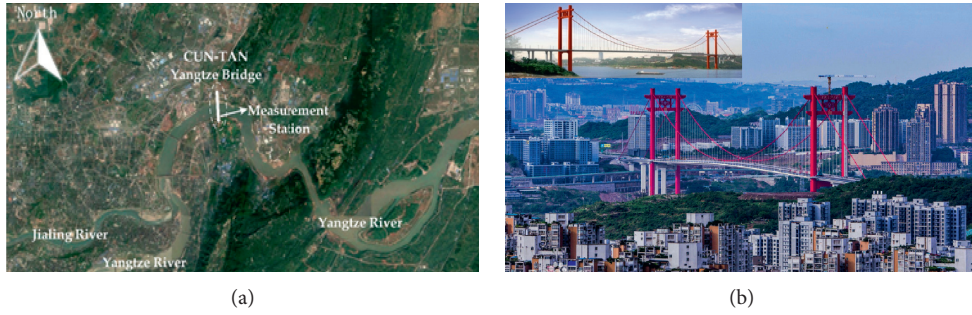
FIGURE 1: (a) Geographical location of the bridge. (b) Overlooking view of the bridge.
