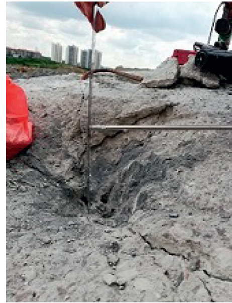
FIGURE 6: Cutting depth measurement.
