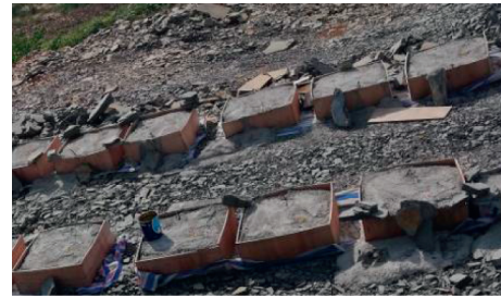
FIGURE 3: Forming of concrete specimens.
