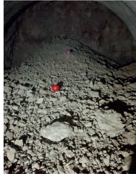
FIGURE 27: The picture of tunnel blasting effect.
