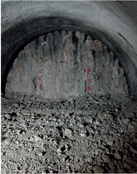
FIGURE 26: Layout of site blast holes.
