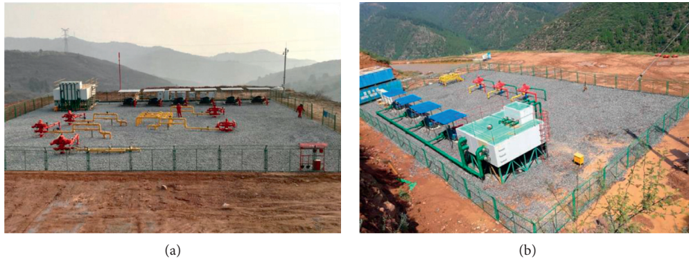
FIGURE 2: Surface layout of CBM well site.
