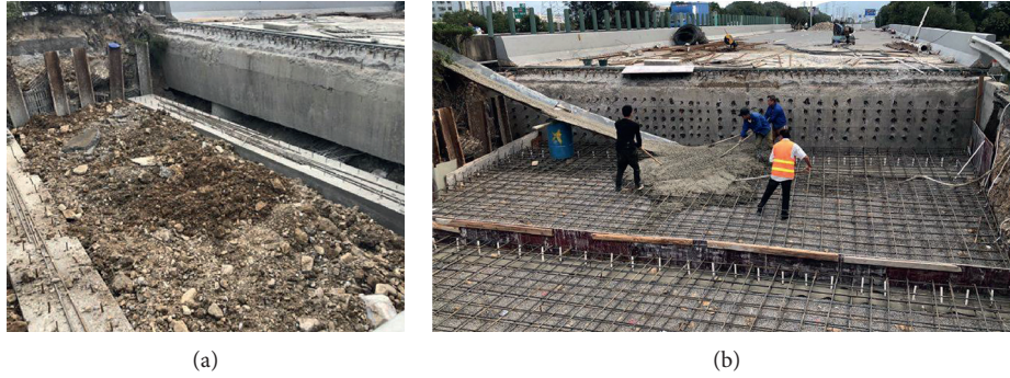
FIGURE 2: Construction site lower partition slab construction picture.
