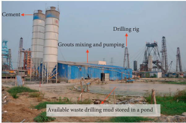
FIGURE 8: Grouting using the waste drilling mud.
